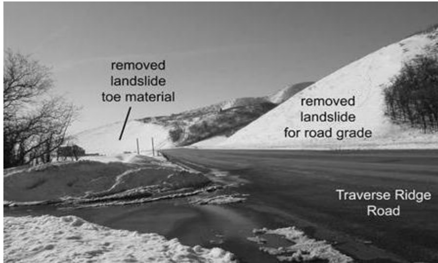
Figure 10. Southwest view along Traverse Ridge Road, near the landslide 40 -landslide B area. Road construction through the region has removed a significant amount of landslide material. Homes have been built in the down slope region.
