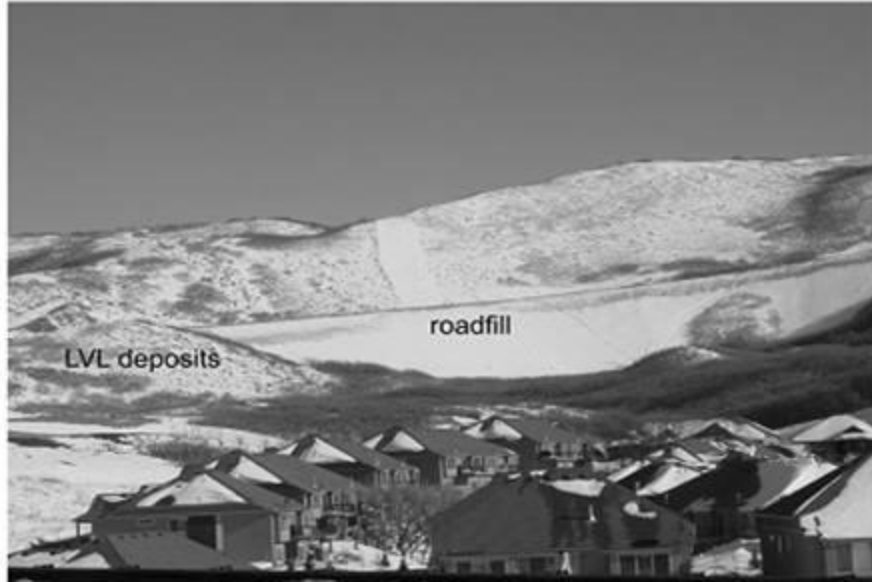
Figure 8. A -- Photograph showing where LVL deposits were removed to construct the primary connector road to the mountainous region. Construction of Traverse Ridge Road involved extensive modification of the landscape. Deposits were removed from the toe area and there was extensive grading of topography within the LVL zone of accumulation. B -- Looking east from the "valley bowl" within the LVL zone of accumulation, towards the Traverse Ridge Road, which is the main access road that snakes up the mountain at a 10% grade. Road building has eroded the lateral margins of the slide deposit. Hummocky terrain is present between the houses and the road fill.
