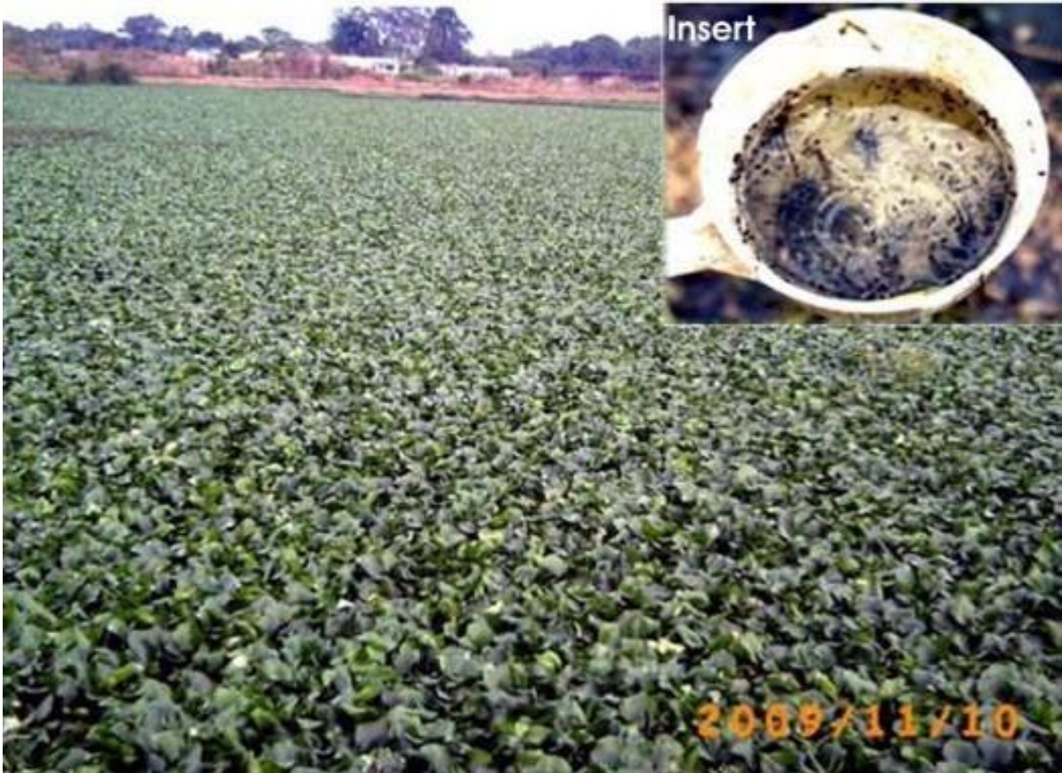
Figure 2. Proliferation of the aquatic vegetation (hyacinth) in the sewage treatment ponds. The insert is a scoop showing the presence of larvae (appearing as dark spots) in the pond-water. Source: Investigator, Nkhuwa DCN.
