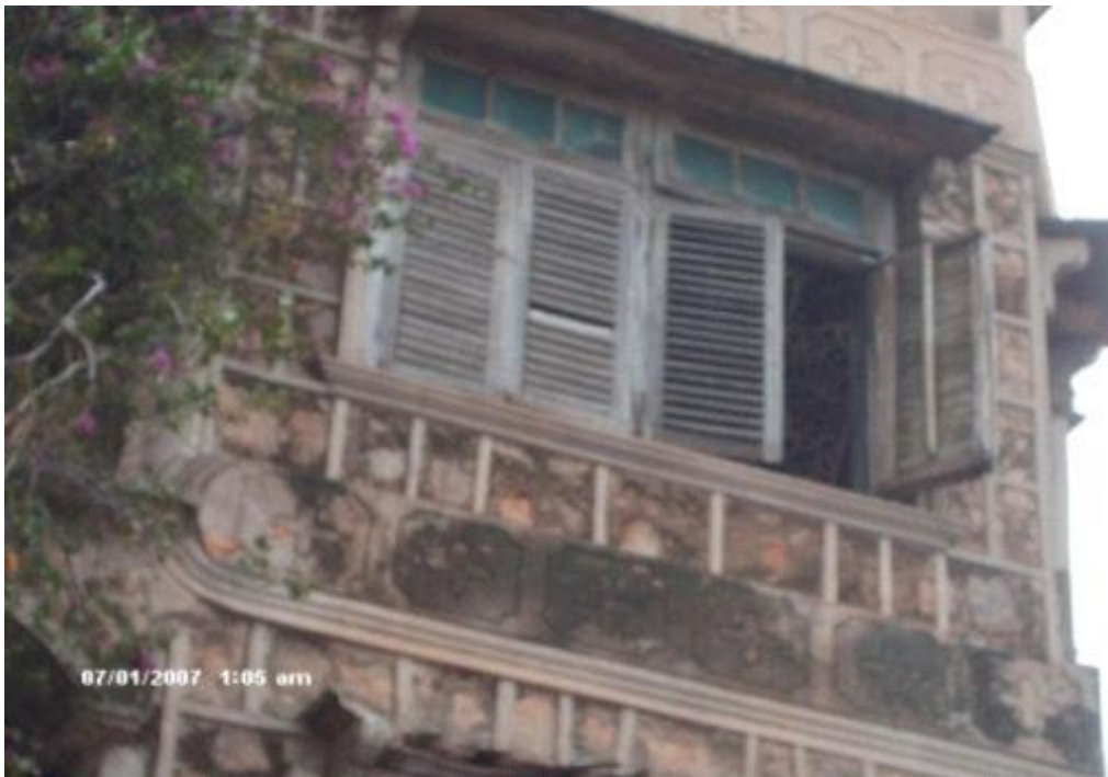
Figure 5. The stone rubble walls of Sussan Wenger's Building, Osogbo, Nigeria.
