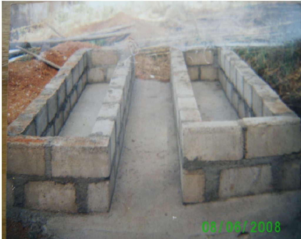
Figure 5. Construction of an anaerobic digester.
