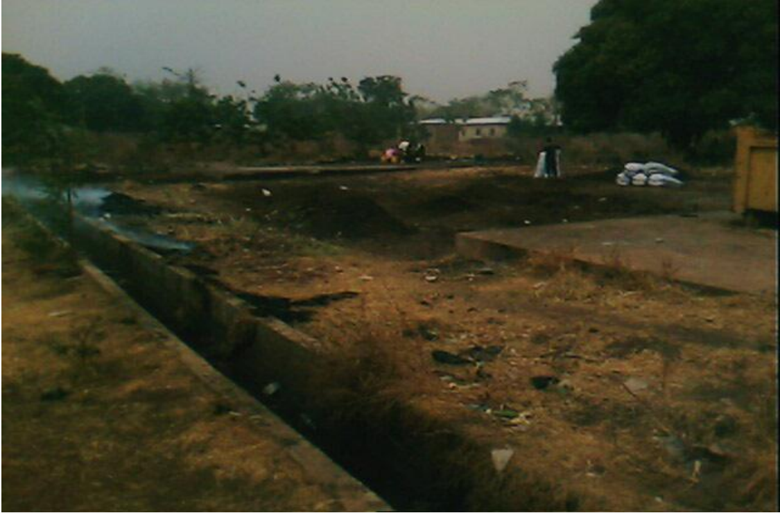
Figure 3. External drain carrying effluent towards community.
