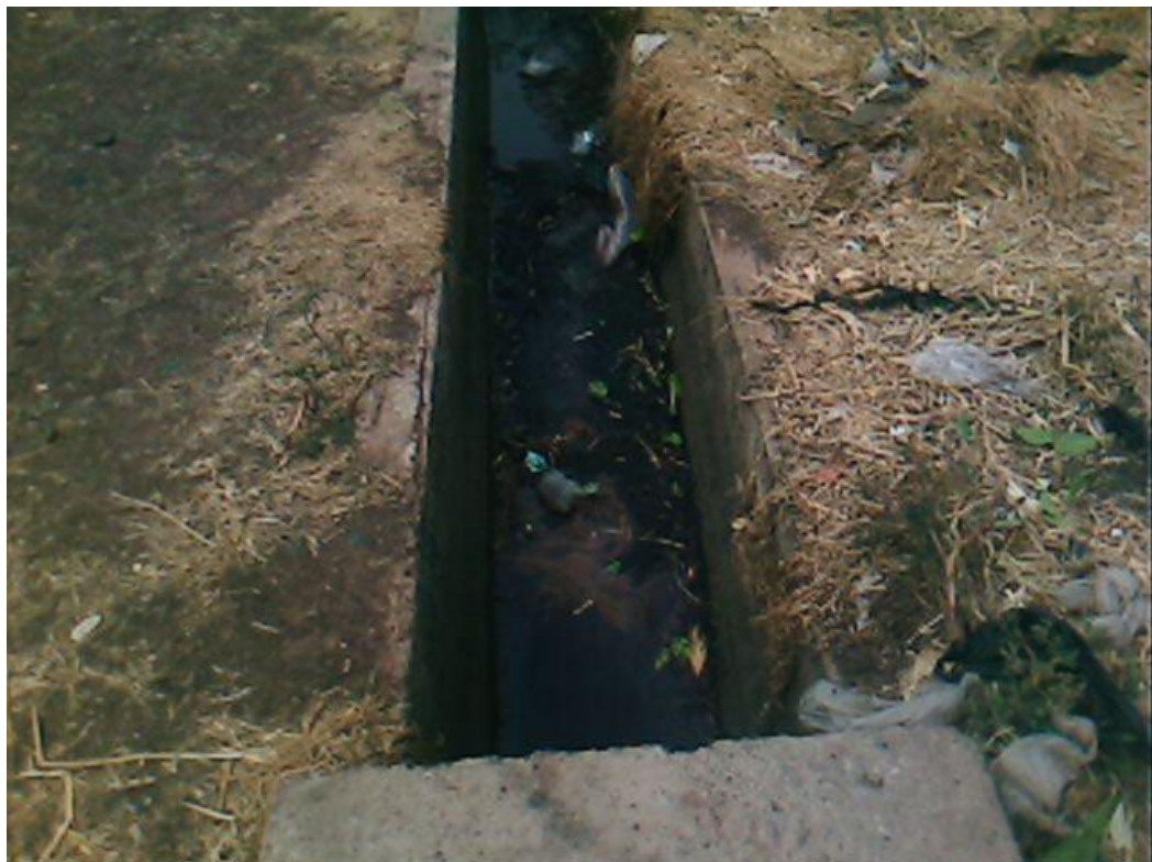
Figure 2. External drain carrying effluent from abattoir.
