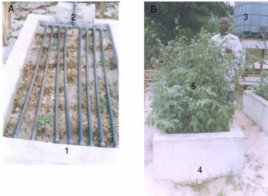
Figure 1. A view of the vertical completely drained constructed wetland planted with Corchorus oliterius . 1: the bed structure in cement brick; 2: irrigation device in PVC; 3: wastewater stocking tank; 4: filtrate drain in PVC; 5: C. oliterius after three months on the bed. A: A view of a bed just after planting the young C. oliterius . B: A view of the planting bed with C. oliterius after three months.
